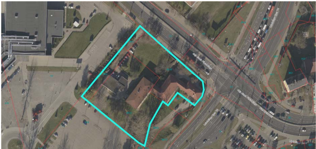
AERIAL VIEW OF THE PROPERTY
